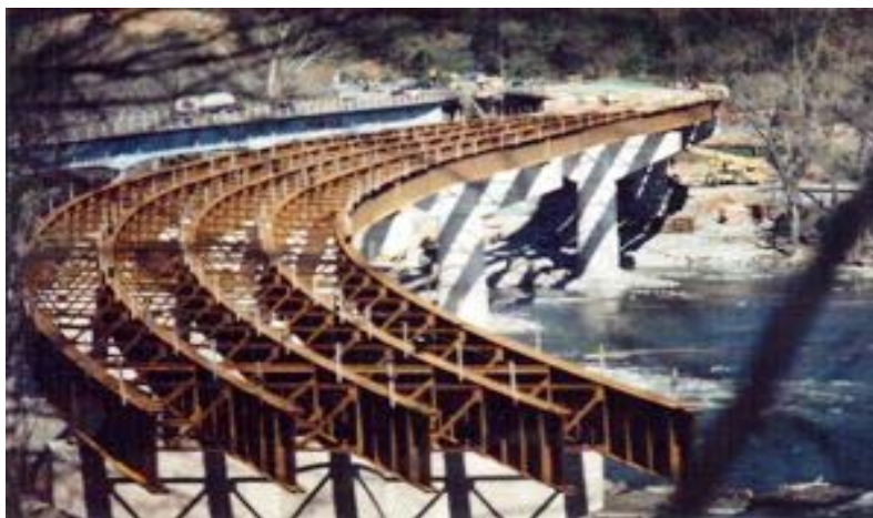
Figure 4.1-1. A Curved Steel I-girder Bridge Similar to the Studied Bridges
